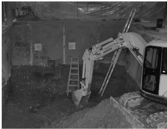
Figure 13: Excavation of Final Phase
