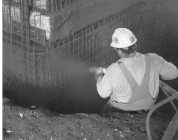
Figure 12. Shotcrete Application
