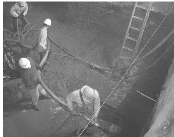
Figure 14: Final Shotcrete Application
