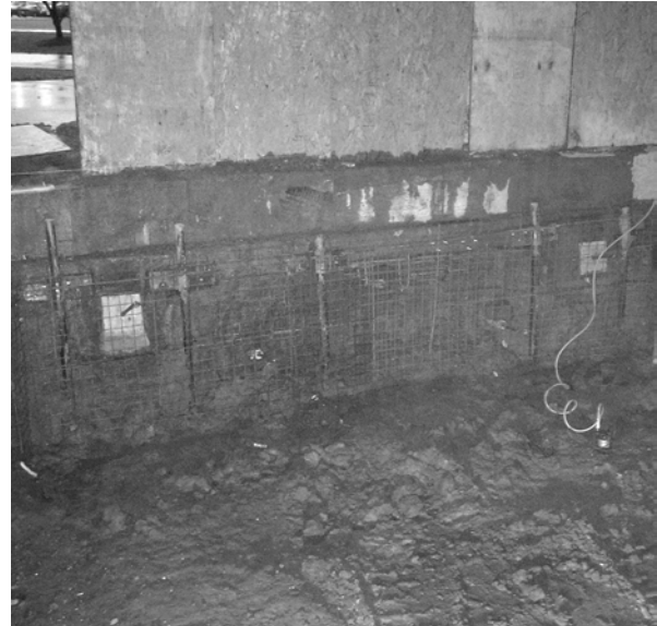
Figure 10. Reinforcing Steel Placement
