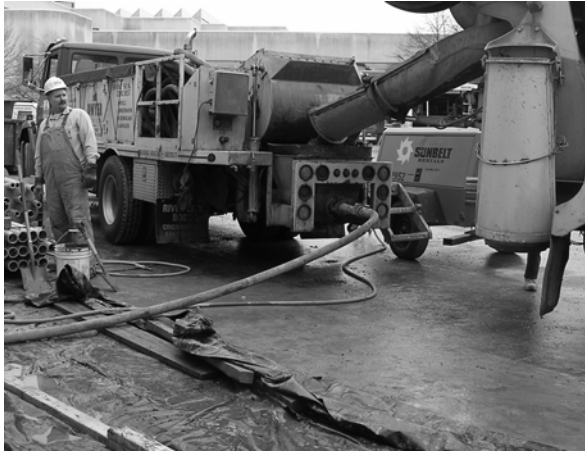
Figure 11. Shotcrete Operations
