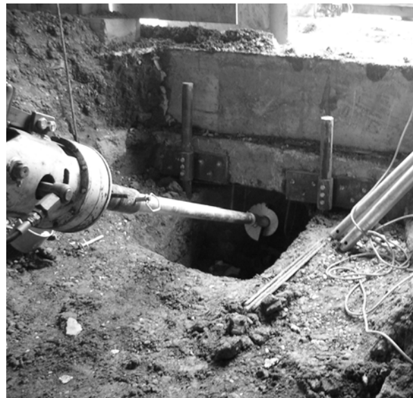
Figure 8: Tieback Installation
