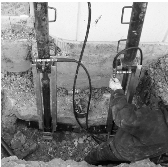
Figure 7: Push Pier Installation
