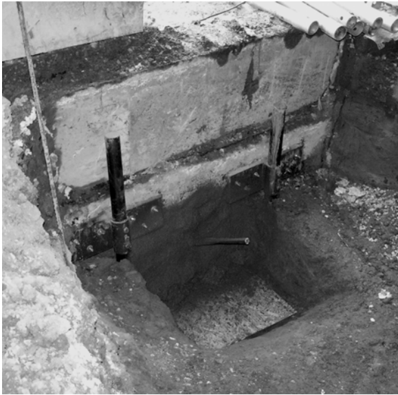
Figure 9. Completed Tieback Haunch
